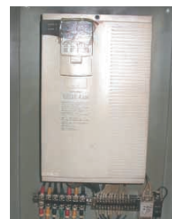
Inverter that controls pump motors
