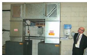
Using air compressor exhaust heat
