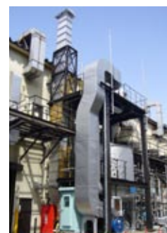
Picture 1: Regenerative thermal oxidizer for gas emissions
