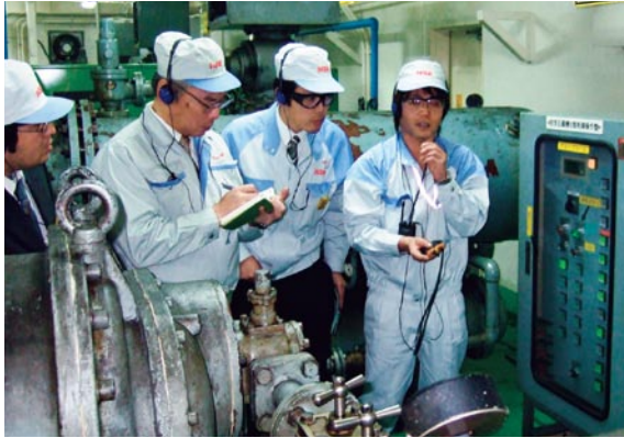
Photo 1: Compressor Working Group in the field
