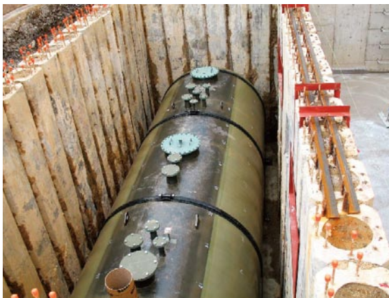
Photo 1: Upgrade to a double hull structure for an underground tank
