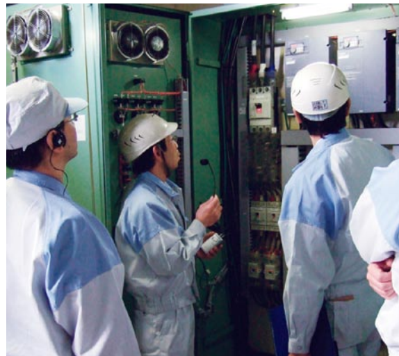
Photo 3: Water Supply Pumps and Ventilation Fans Working Group in the field
