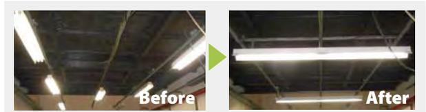
Photo 3: Measure to save energy used by lighting equipment at NSK Brasil Ltda., Suzano Plant
