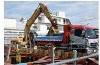
Photo 2: Soil contamination countermeasure work at the former site of the Tamagawa Plant
